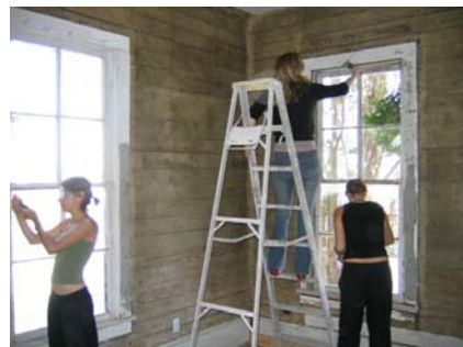
Volunteers Paint the New Offices
