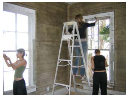
Volunteers Paint the New Offices
